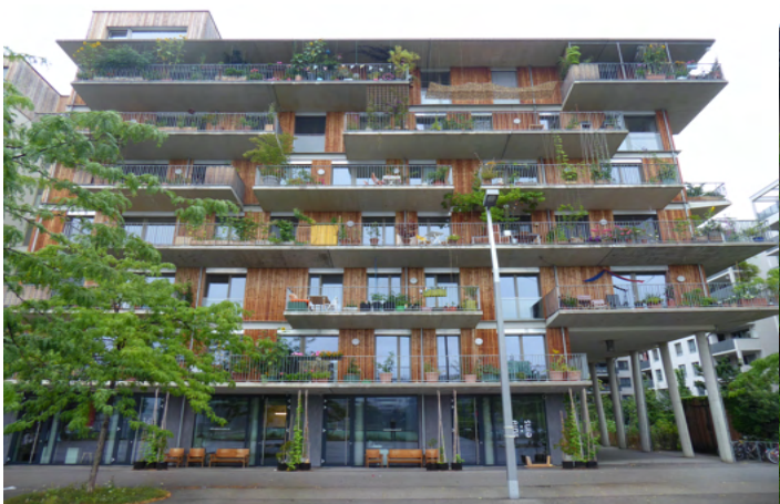
Wohnprojekt Wien housing cooperative in Vienna
